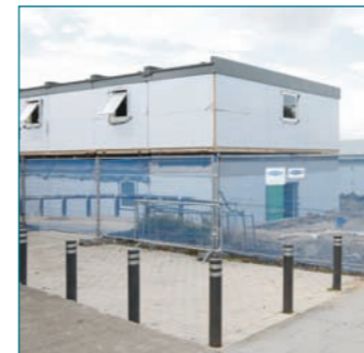
The new Health Centre site on Ponteland Road
