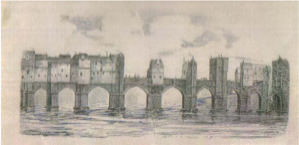
View of the Medieval Bridge from the east
